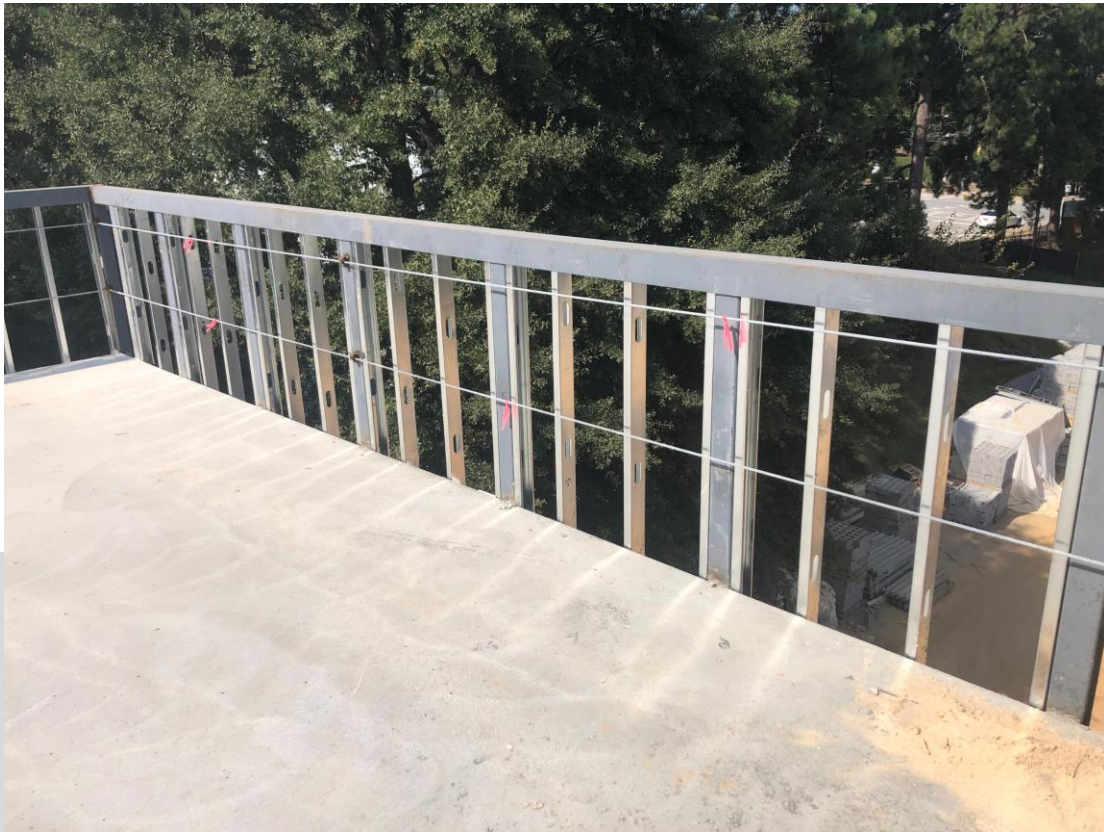
Exterior Framing Complete at New Patio
