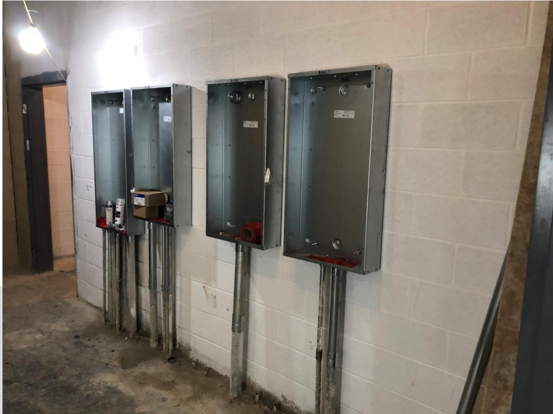
New Panels Installed at Main Electrical Room
