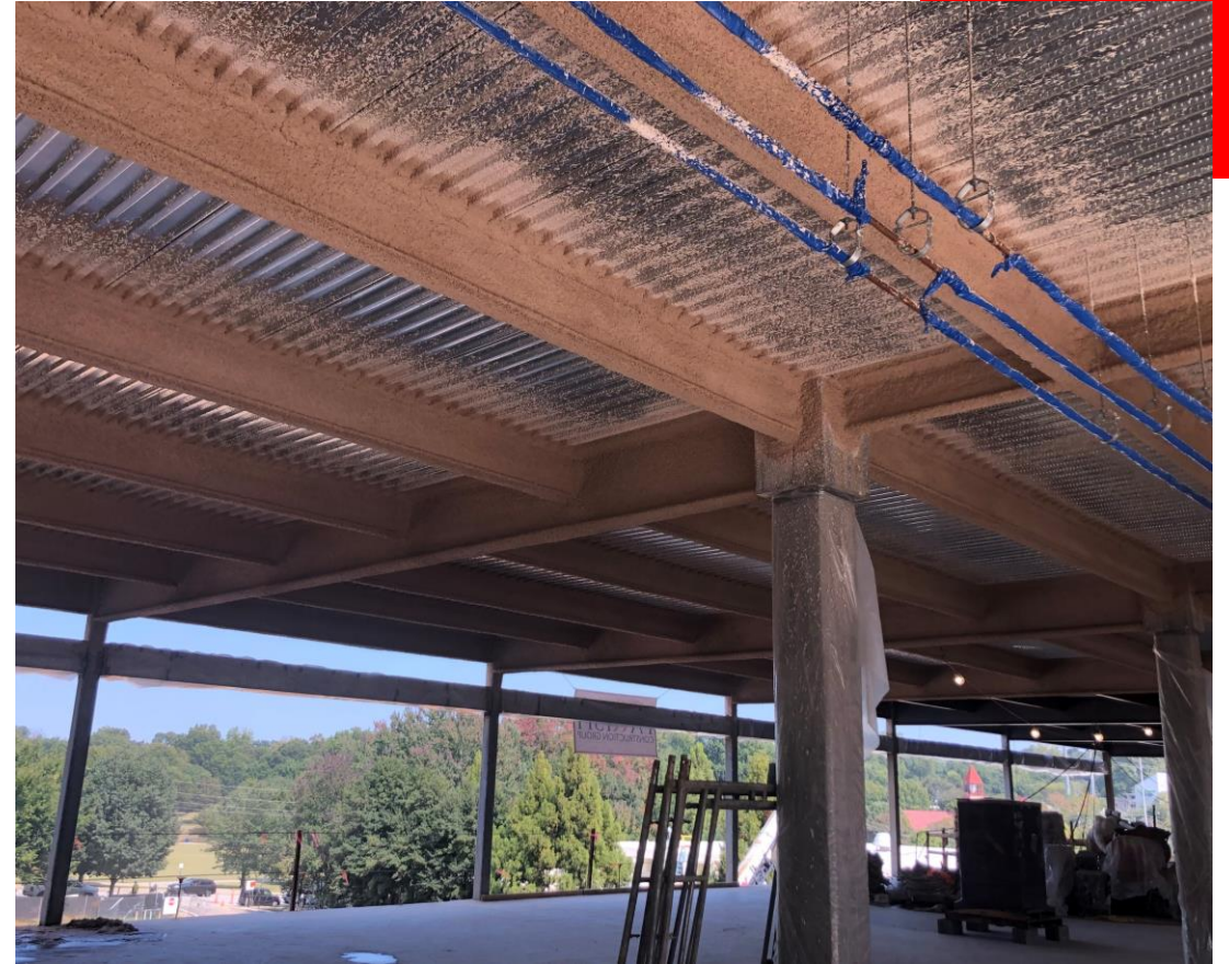
Third Floor Fireproofing Completed
