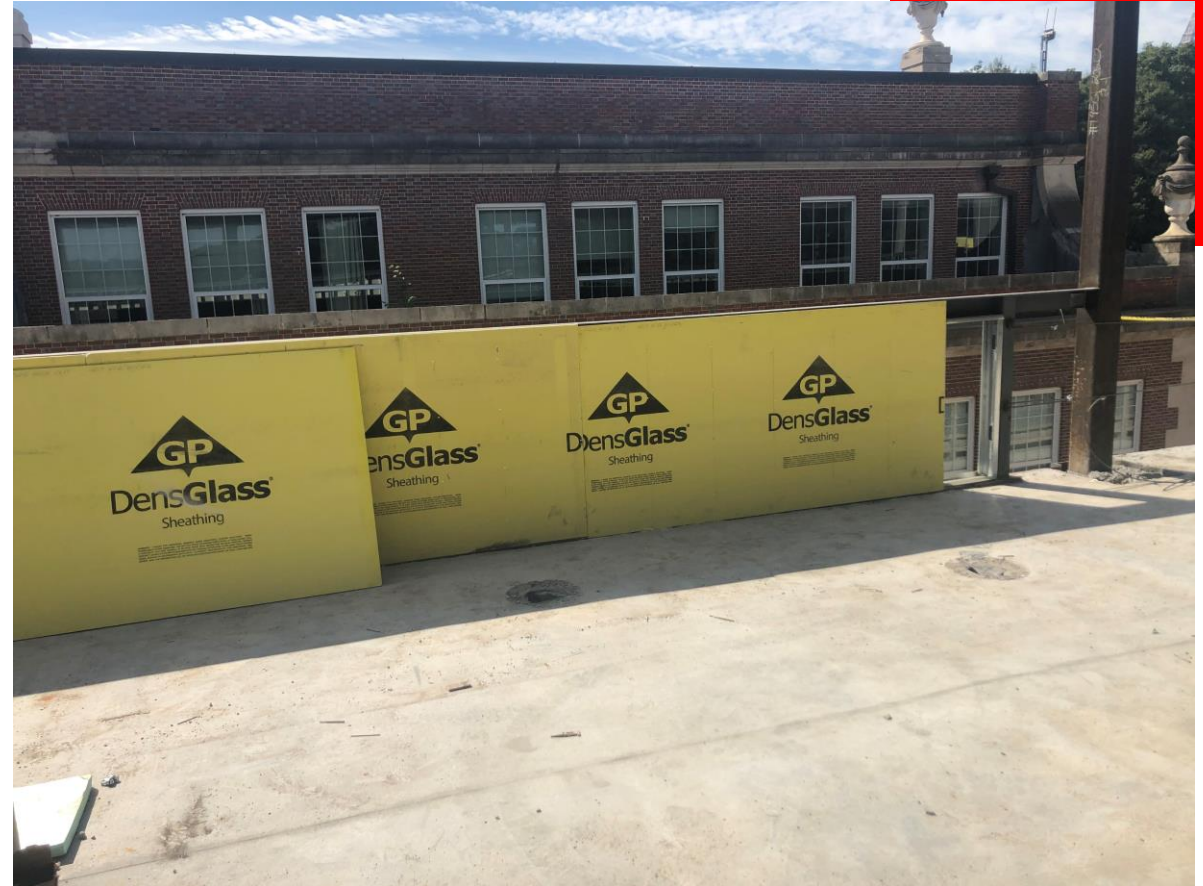
Sheathing Installed at New Addition South Patio
