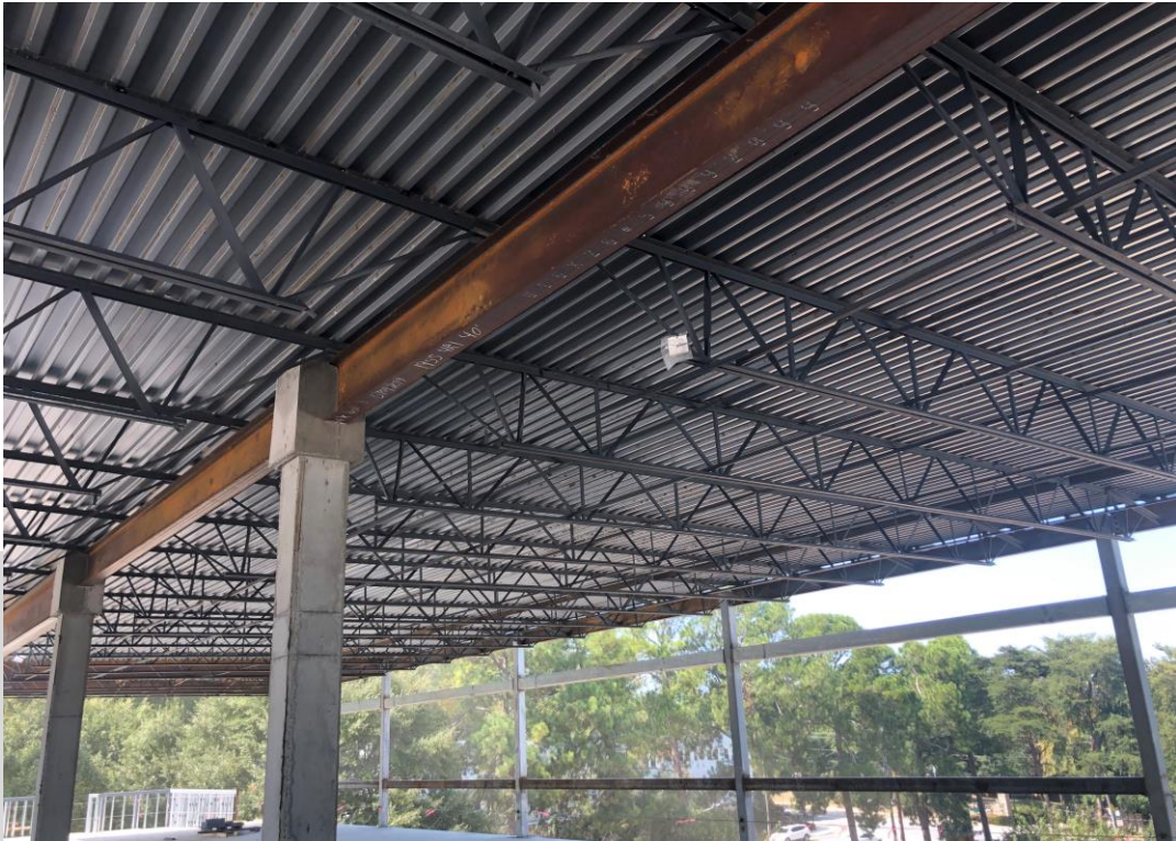
Roof Decking Installed
